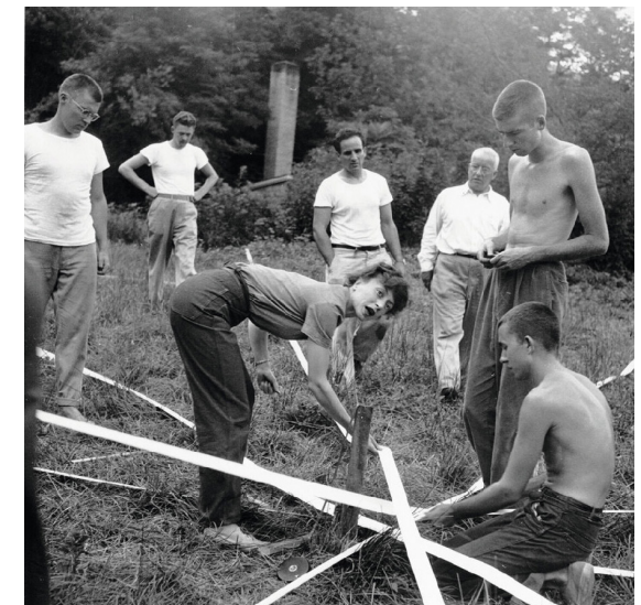
Elaine de Kooning (centre) assembles Buckminster Fuller's Venetian-blind-strip dome at Black Mountain College, 1948.
